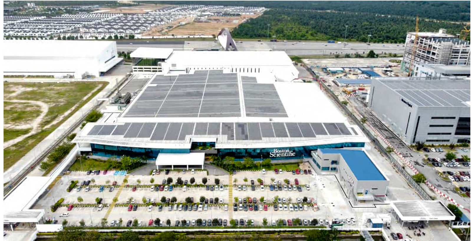
In 2023, we completed installation of solar panels in our Penang manufacturing site. This is currently our largest solar installation.
